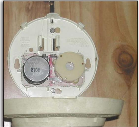
The existence and reason for the missing battery in this smoke alarm should be documented in the investigator's report.
