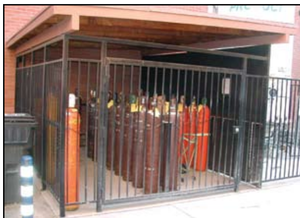
With two enclosed sides, this example should be classified as “indoor storage.”
