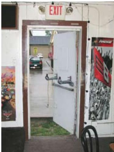
This homemade security system compromises the required egress width.
