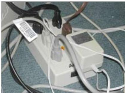
Wattage ratings usually can be obtained from the electrical nameplate on an appliance. In the United States and Canada, branch circuit voltage nominally is 120 or 240 volts. Dividing watts by volts will give you a relative idea if the branch circuit is “overloaded,” that is, if it has too much current draw for the overcurrent protection.
