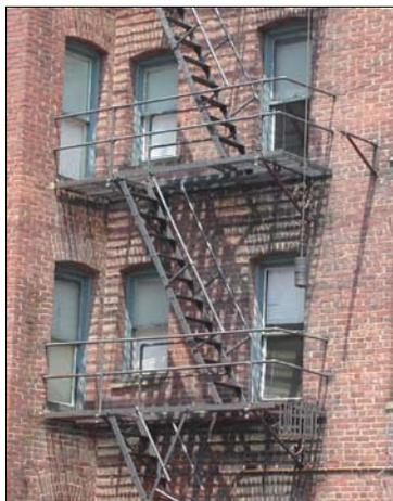
Openings near the fire escape should be protected with approved fire door or fire window assemblies having a minimum 45-minute fire-resistance rating. The distance and arrangement of opening protectives varies by the different codes.
