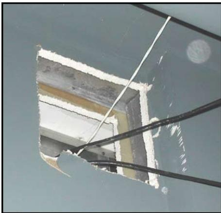
This compromised fire-rated wall assembly should be repaired to meet the building code requirements for fire resistance.
