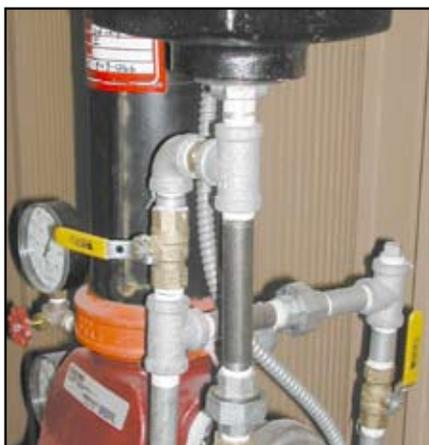
The quarter-turn alarm line valves have been left in the “out-of-service” position on this wet-pipe alarm check valve with retard chamber.
