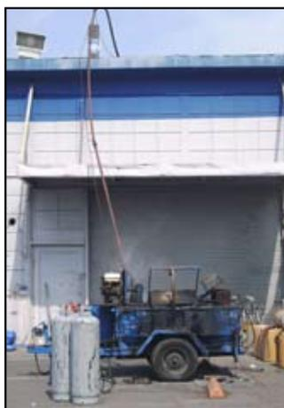
This mobile asphalt kettle should have at least one fire extinguisher nearby, and the cylinders should be secured from falling.
