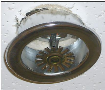
The escutcheon for this recessed sprinkler must be part of a listed sprinkler assembly so if it loosens it won't interfere with water spray.
