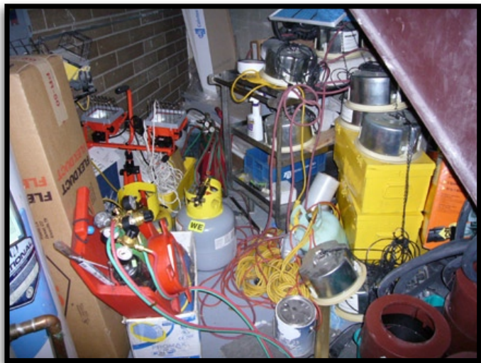
The variety of hazards in this photograph are almost too numerous to mention.
