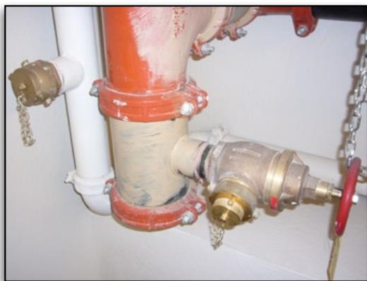
The threaded inlet connection on the left provides a drain for testing the pressure regulating hose outlet.
