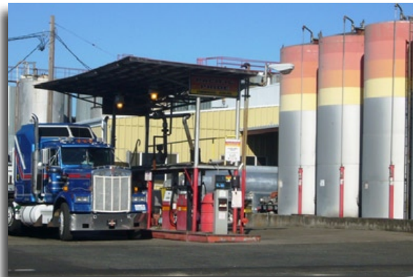
This bulk transfer site must meet the fire code requirements for flammable liquid safety.
