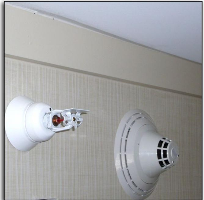
The sprinkler and smoke detector must be located below the ceiling in accordance with listing and code requirements.
