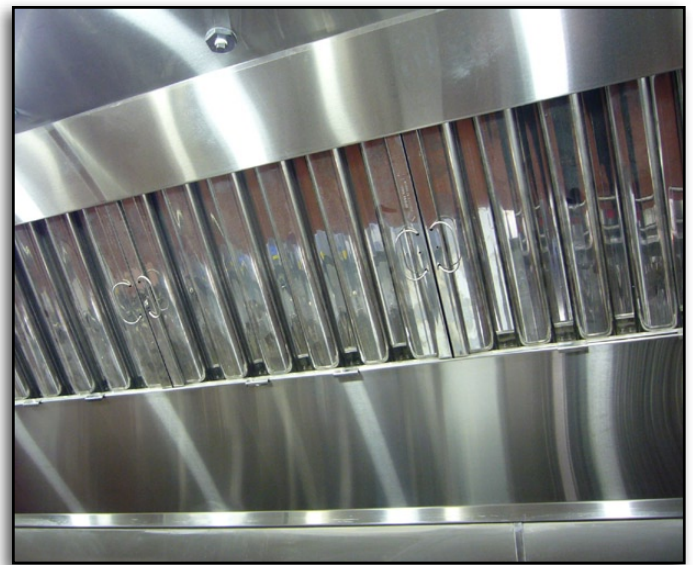
These “baffle-style” grease filters meet listing requirements for commercial cooking ventilation systems.
