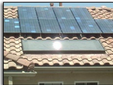
Photo courtesy California State Fire Marshals Office. This rooftop is equipped with both photovoltaic (upper) and water heating solar panels.
