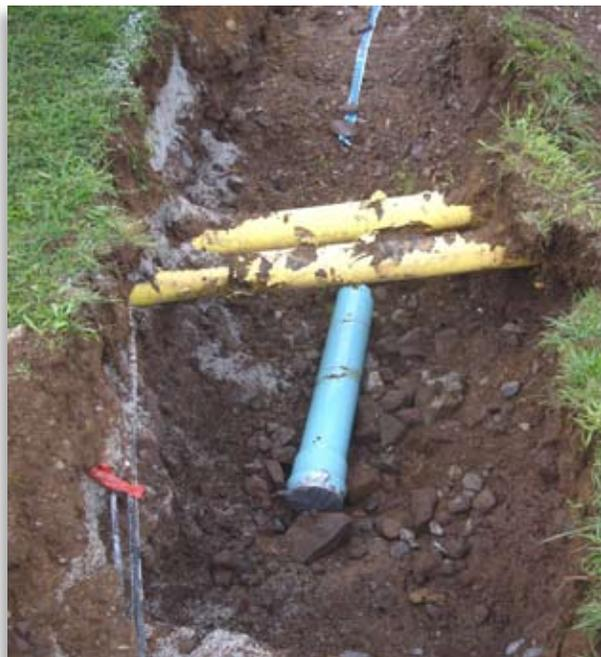
This trench should be deep enough that the water main will not be exposed to freezing temperatures.
