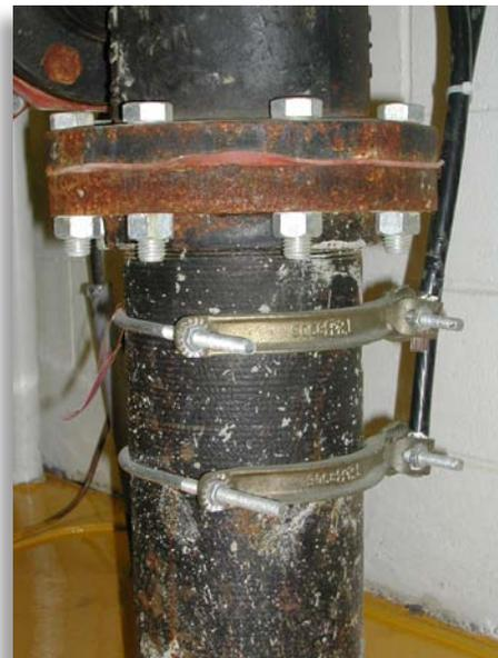
This sprinkler riser is appropriately bonded to the metal building in which it is located.
