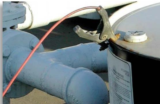
This bonding clip connects to another container to remove the electrical potential.
