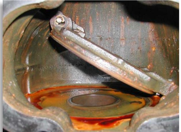
This open dry pipe valve housing illustrates the size difference between the incoming waterway and the upper valve surface.
