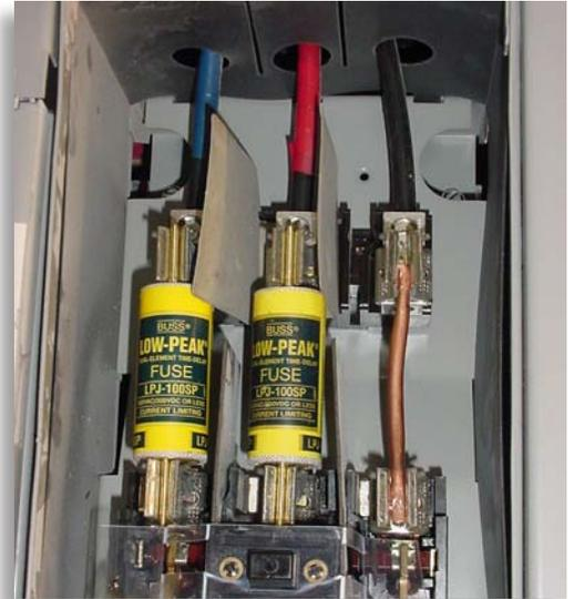
A piece of copper tube has been inserted in the fuse box creating an illegal and dangerous hazard. Photo courtesy Keith Heckler, Rockville Fire Department, MD.
