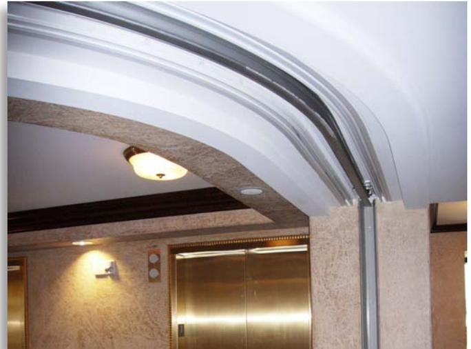
The curved track on the ceiling guides a motorized fire door used to create an elevator lobby.
