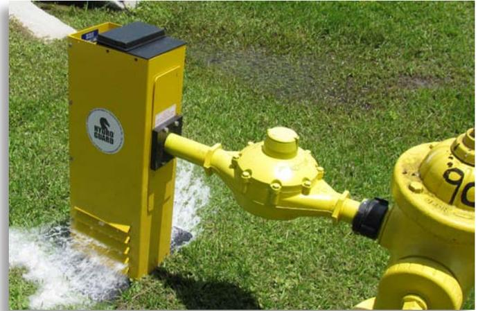
Automatic water system flushing device attached to hydrant showing water flush cycle. Photo courtesy of Hydro-Guard®.
