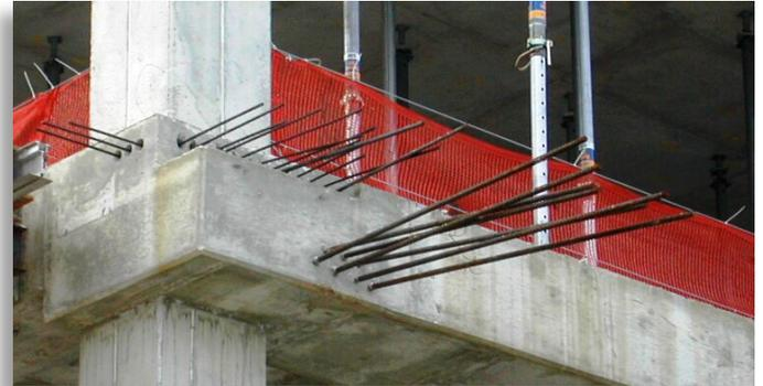
These posttensioning rods used in concrete construction add strength, but do not affect the concrete's stiffness.
