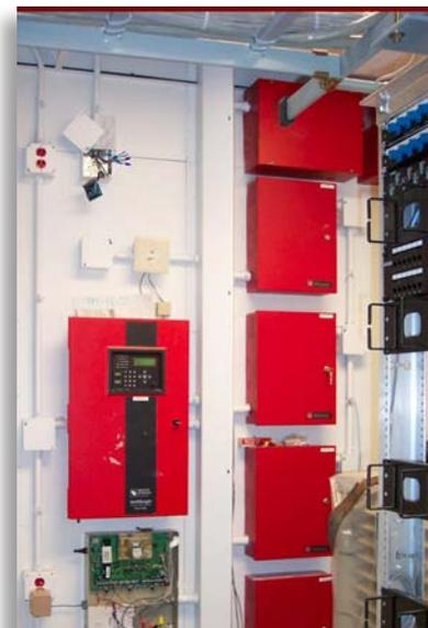
This fire alarm control panel is designed to transmit a signal to an offpremise reporting facility.
