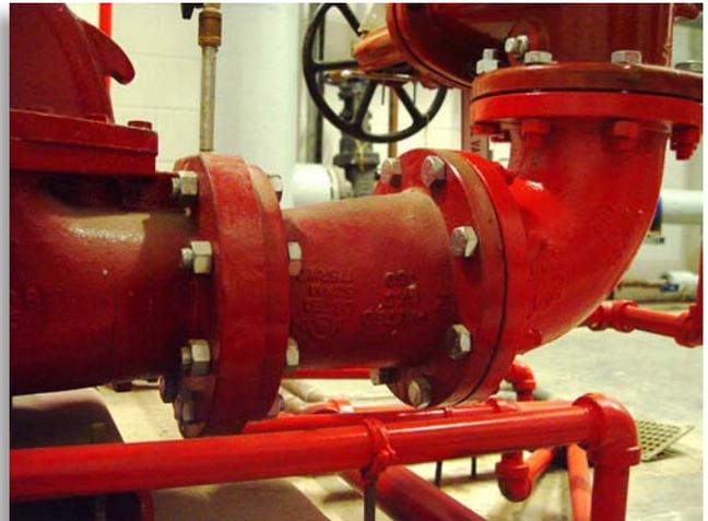
This eccentric reducer is installed correctly with the “flat side” down in a top-feed configuration. Photo courtesy Keith Heckler, P.E., Rockville Fire Department, Maryland.
