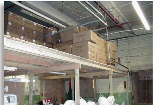
This "add on" mezzanine increases storage capacity, but requires automatic sprinkler protection beneath it. Photo courtesy of Martin M. King, West Allis, WI.
