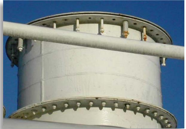
The long bolts at the top of this liquid storage tank manway should never be tightened.
