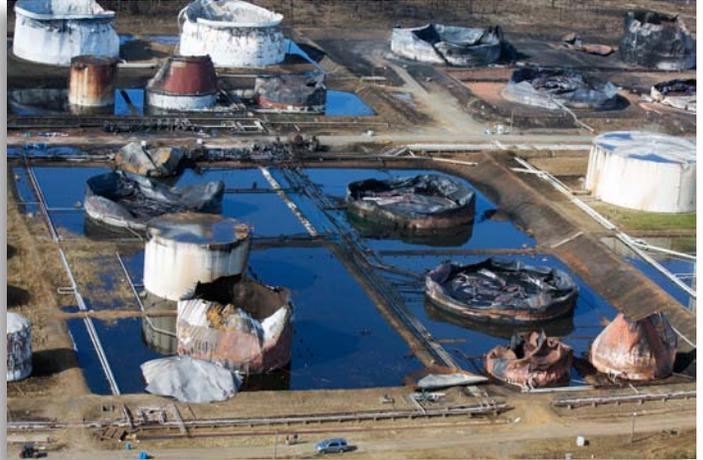
This postincident photograph illustrates the importance of spill control around aboveground flammable and combustible liquid tanks.
