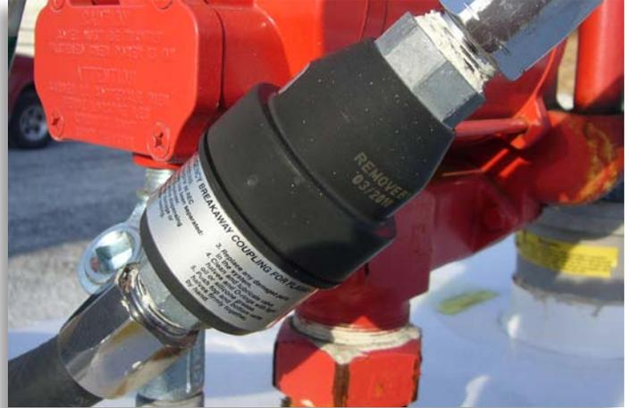
This breakaway device is intended to stop fuel flow in the event the dispenser hose is pulled from its connections.
