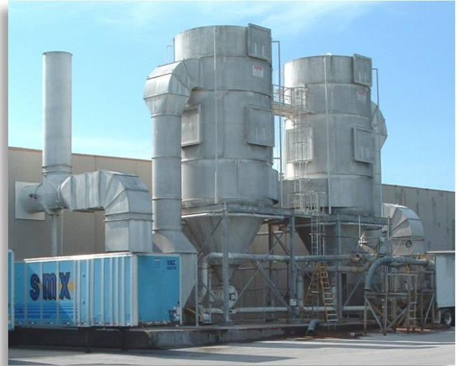
The square devices on these cyclone collectors are explosion vents to relieve deflagration pressure in the dust collection system.
