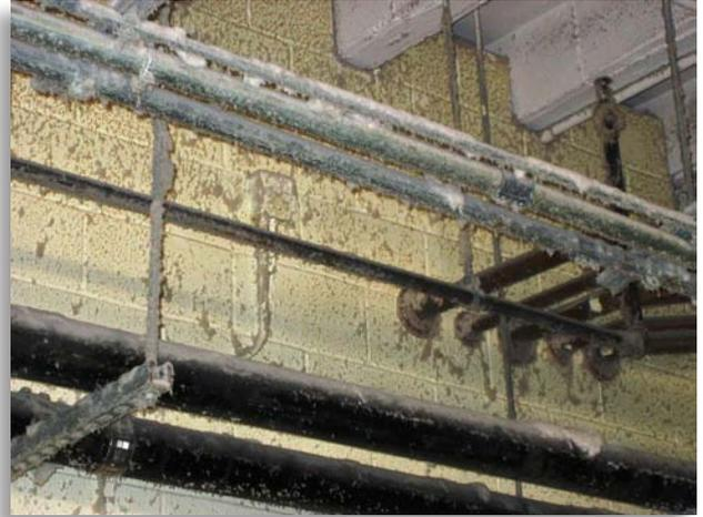
The accumulation of highly combustible lint in this commercial laundromat should cause the inspector to review the electrical classified location requirements.
