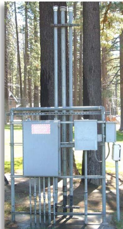
The area around these underground gasoline tank vents must be classified because flammable vapors are heavier than air.
