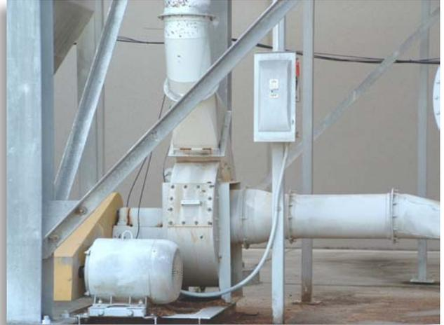
Electrical equipment around this wood dust collection cyclone should be evaluated for compliance with Class II, Group G hazardous (classified) locations.
