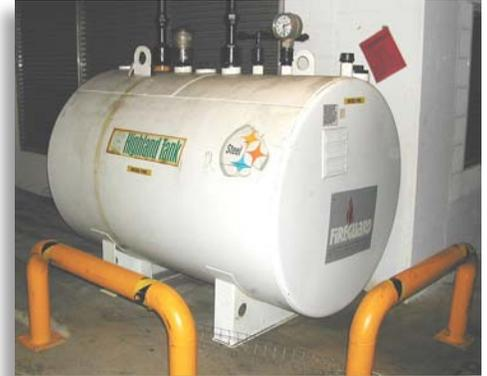
This protected aboveground tank in a parking garage contains diesel fuel, also known as Fuel Oil No. 2.
